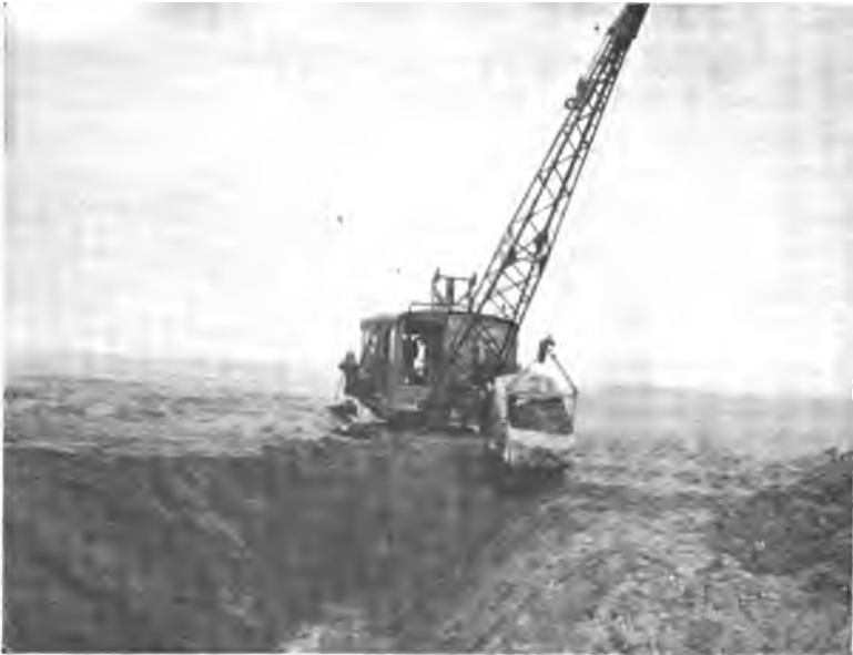
FIG. 62.—Dragline Excavator on Drainage Work, Idaho.
